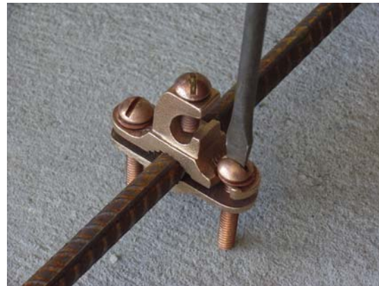
Step 2 – Tighten the fastening screws to ensure a secure connection to the rebar.
