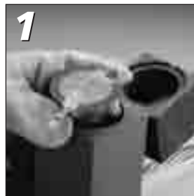
1 Insert CADWELD PLUS package into mould
